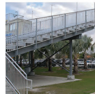
Aluminum bleachers with I-Beam construction, as shown, allow access for ease of maintenance below the bleachers.
