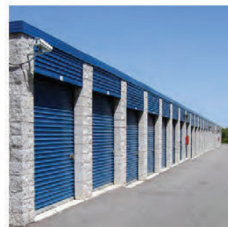
Garage doors allow easy access to linear storage buildings for athletic equipment, buildings and ground maintenance materials. The buildings back wall provides a barrier between the city sidewalk and the stadium.
